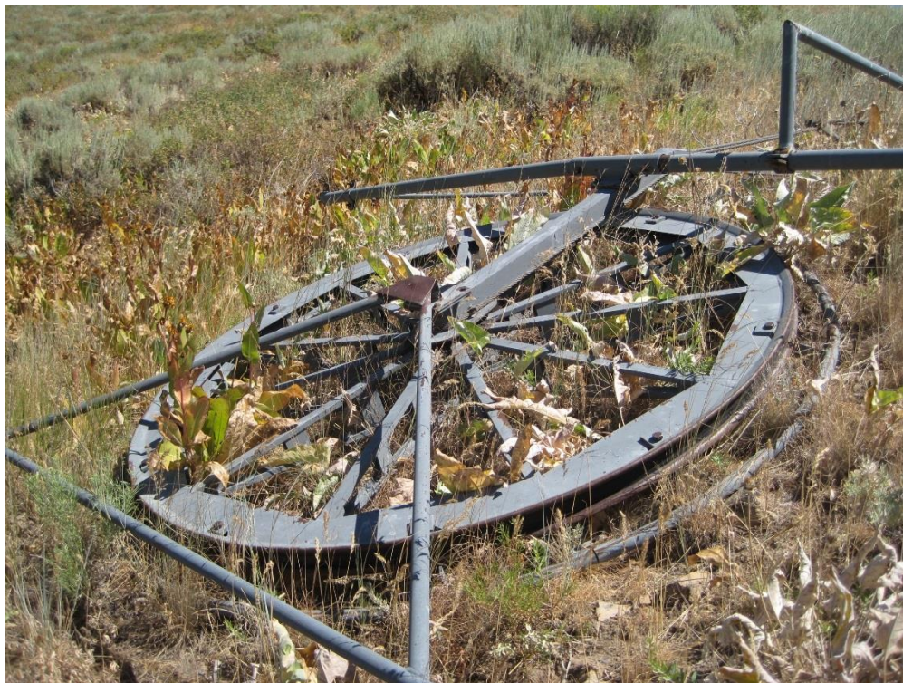
64. Poma Platter Surface Lift (#26), abandoned summit station bull wheel structure, August 2016
