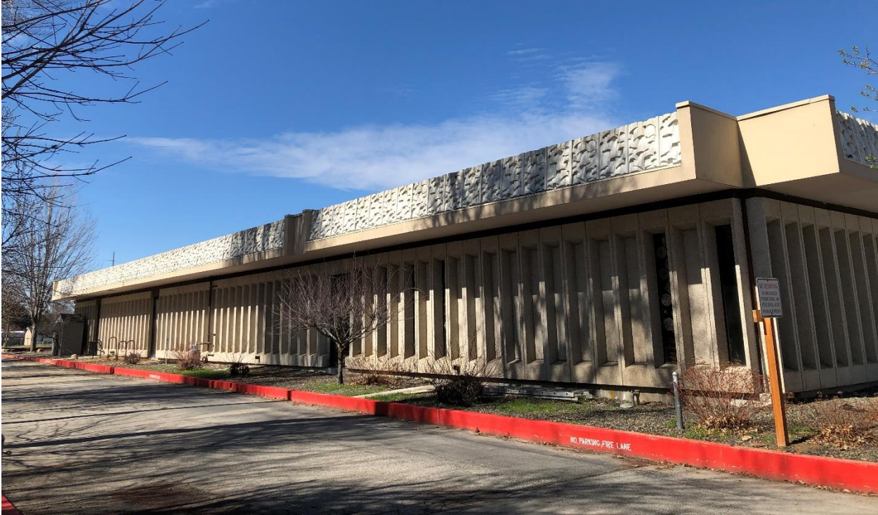
View NW of South Elevation, March 2020
