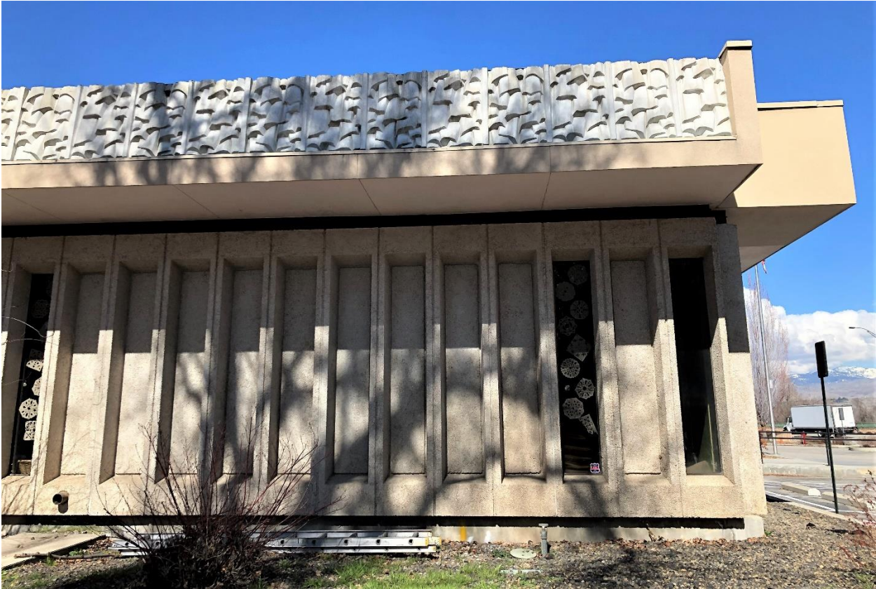
View N of South Elevation, March 2020
