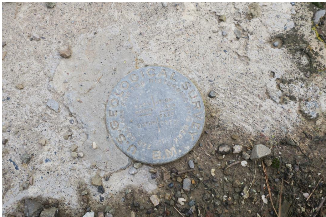
37-005784 , September 2017 Detail view of bench mark on east abutment
