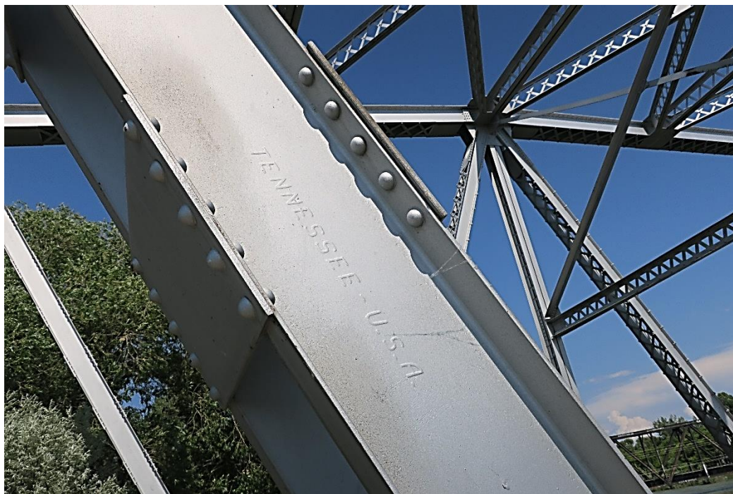
11-005190 (ITD Key #23120), July 2017 View E-NE of typical stock steel marking
