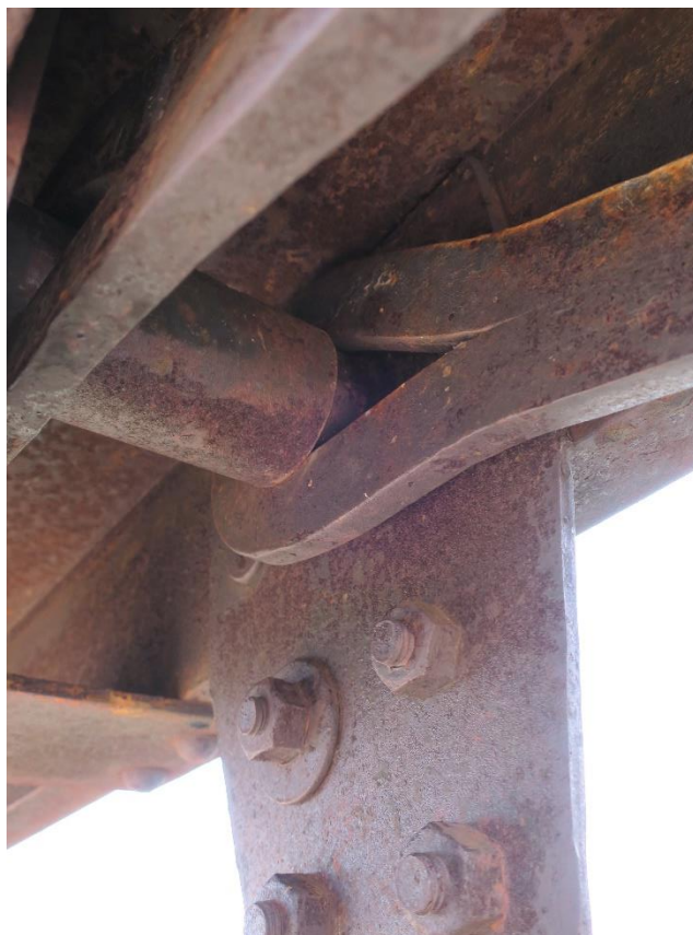
25-005156, May 2017 Detail view of typical pin at upper node
