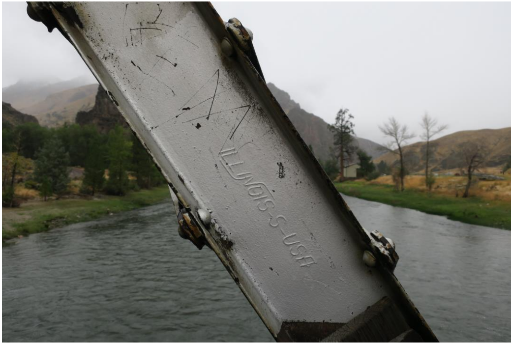
59-004920, September 2017 Detail view of steel manufacturer's mark – "ILLINOIS-S-USA"
