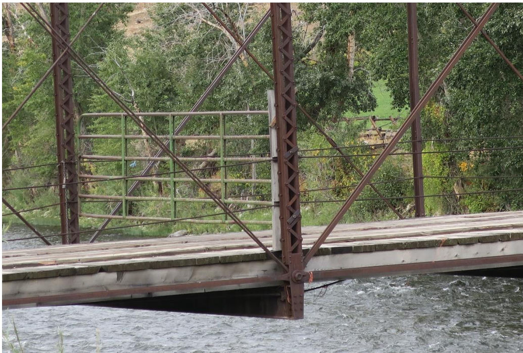
37-004918, September 2017 View SW, typical bottom node
