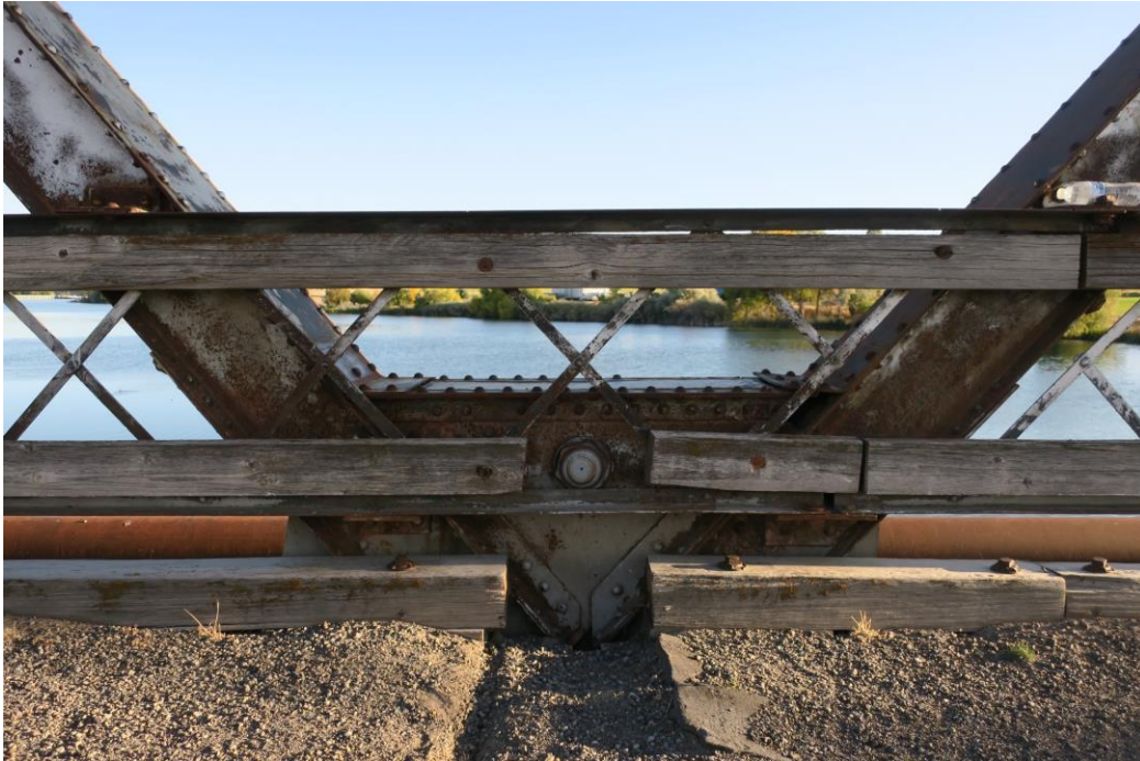
47-005153 (ITD Key #24340), October 2017 View SE of typical bottom node
