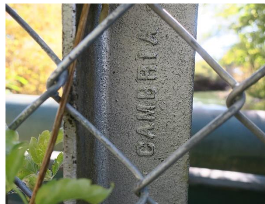
Cambria Iron Works Marking (Little Wood River Warren Truss Bridge (E. 3 rd St.))
