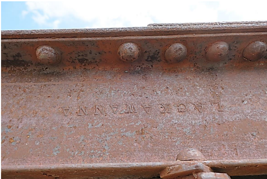
25-005157 , May 2017 Detail view of one of several original stock steel markings
