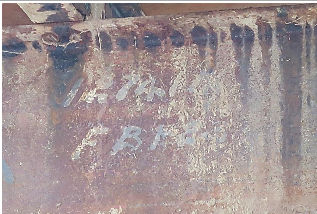
37-005784 , September 2017 Detail view of one of several original construction markings present on floor beams and end posts
