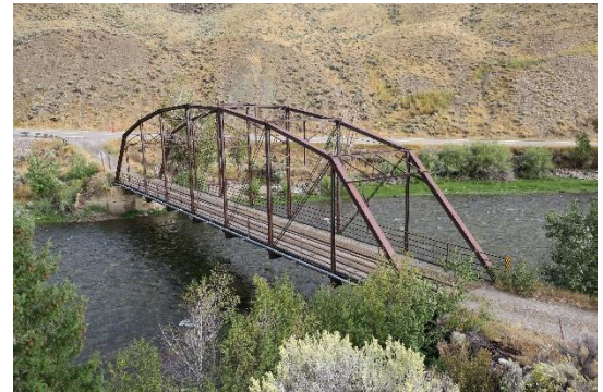
Salmon River Parker Truss Bridge (37-005783; ITD Key# 31650)
