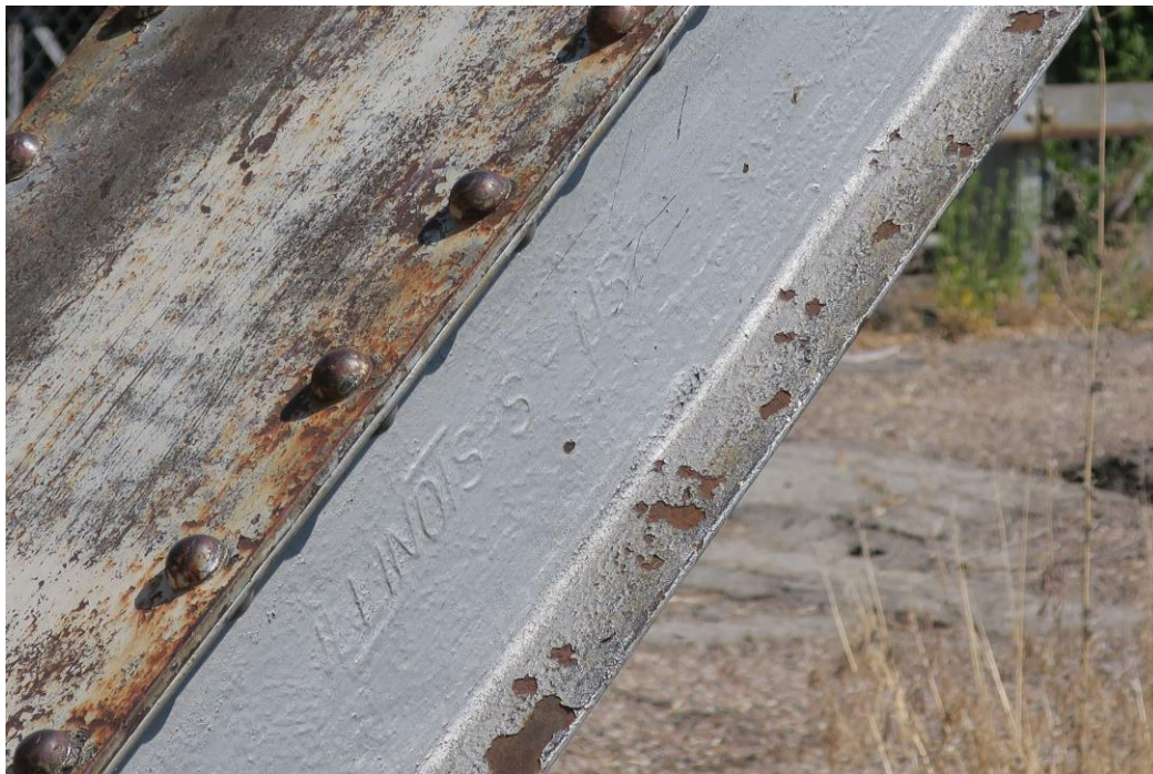
05-005178 (ITD Key #No ITD Key#), July 2017 View of steel manufacturer's mark – "ILLINOIS – S – USA"
