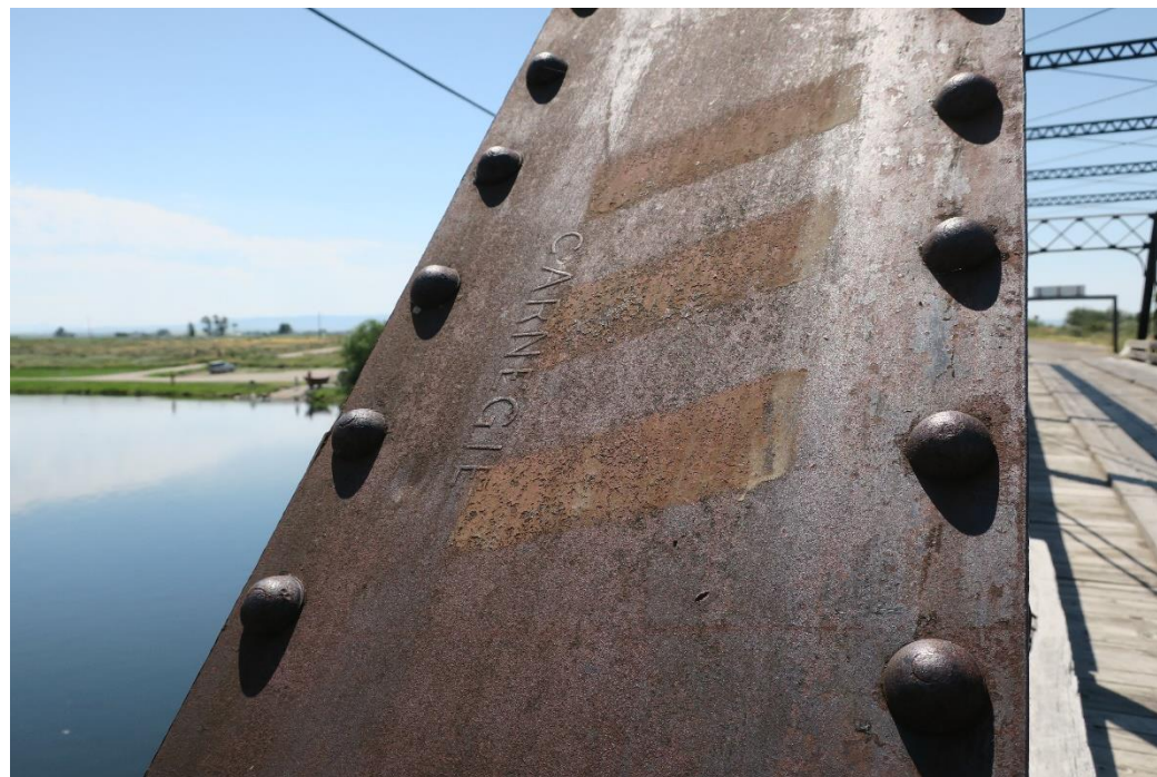
43-005790 , July 2017 Detail view of one of several original stock steel markings
