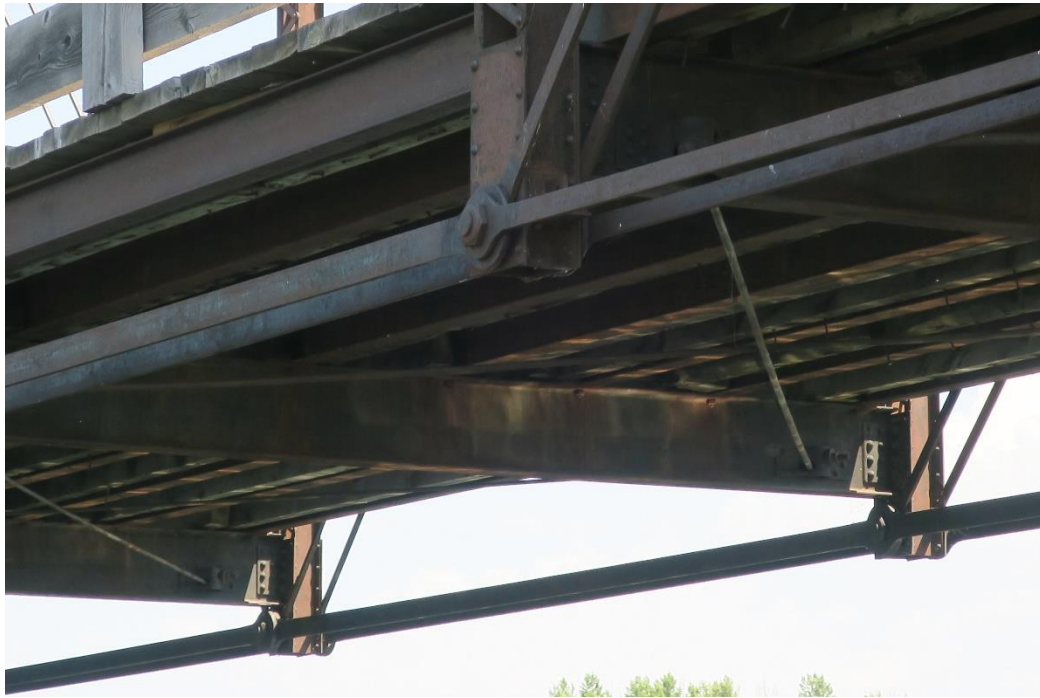
43-005790 , July 2017 Detail view of bottom chords, floor beams, and stringers below deck
