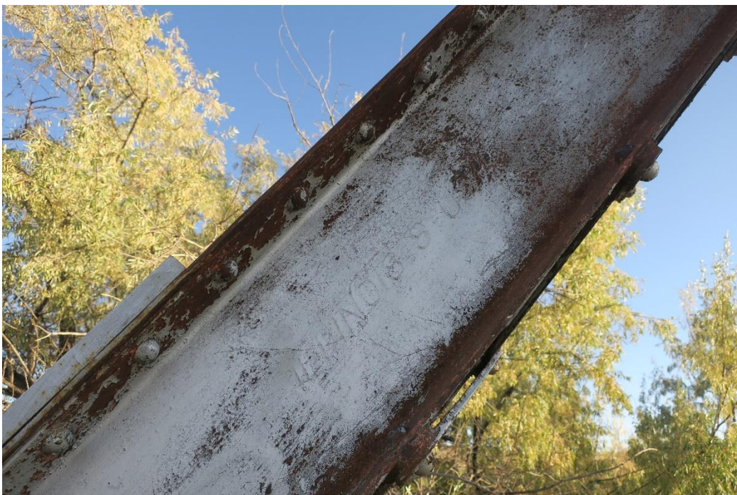
47-005153 (ITD Key #24340), October 2017 View of typical stock steel marking with letters in relief that read, "ILLINOIS - S - USA"
